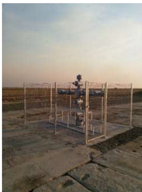
The IMIC-1 Well Head Suspended for Production Testing
