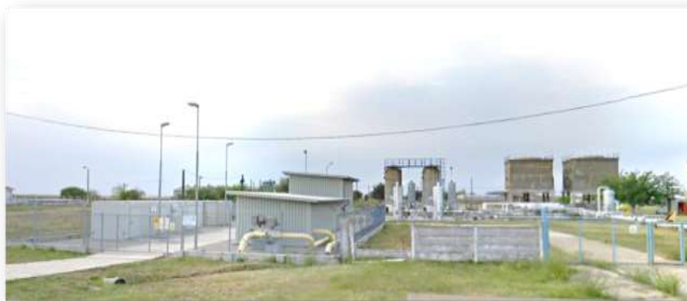
The Calacea Oil & Gas Plant 12 Kms from Ilecea Mica-1 Well
