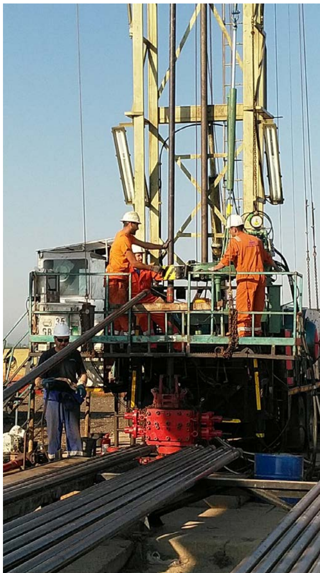
Running production string into IMIC-1 well prior to flow testing
