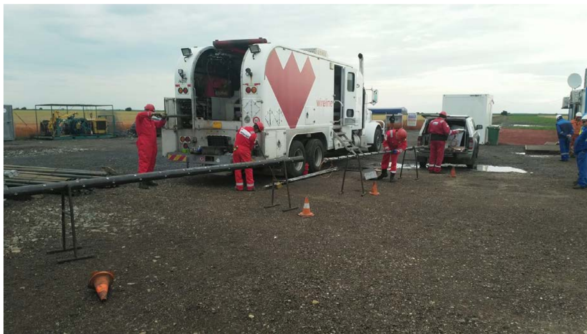
Preparation of perforation equipment prior to running into IMIC-1 well
